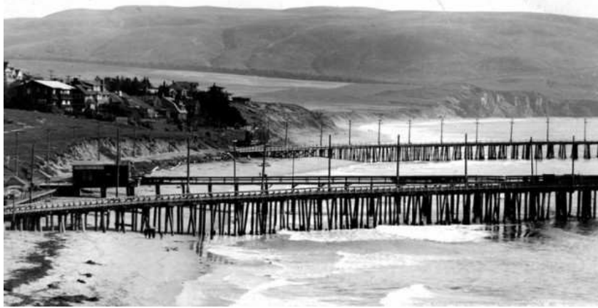
Redondo's Wharf No. 2 and Wharf No. 3
