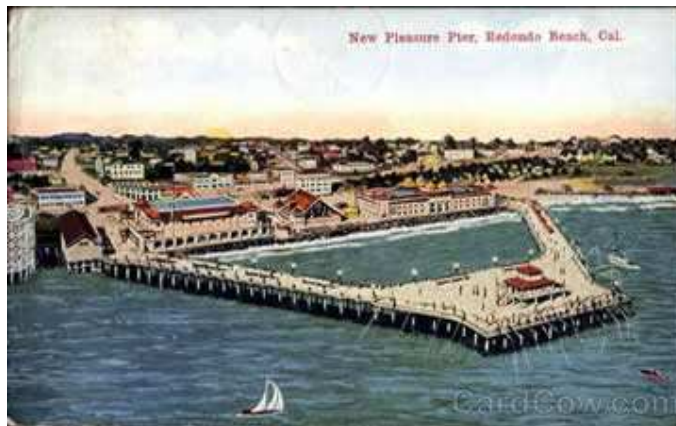
In 1916, a municipal pier referred to as the “endless pier” was constructed in a “V” shape to replace the destroyed Wharf 1. A 450-foot long northern leg began at the former location of the old Wharf No. 1. At the western end of the northerly leg stood a 160-foot x 200-foot platform. From this platform, the Pier headed back to shore just south of the Bathhouse on the 450-foot southern leg.
