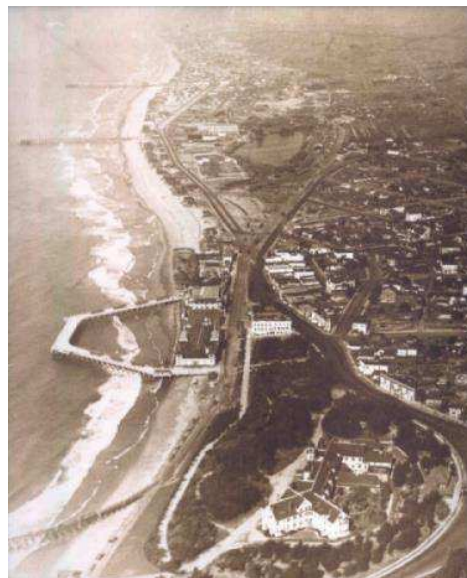
Pleasure Pier and remains of Wharf 2 in front of Hotel Redondo with Hermosa Beach and Manhattan Beach piers at top of picture. Picture probably taken after 1919 storm damaged the pleasure pier and severely damaged Wharf 2
